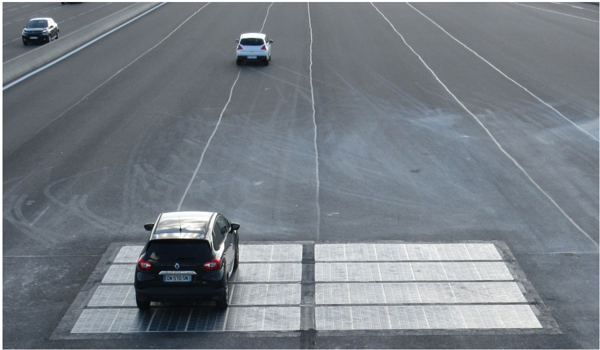
In Saugnac-et-Muret, France, 60m² of Wattway solar panels have been built into the road surface. In ideal sunny conditions, the tiles generate sufficient energy to run the toll gate. © COLAS
